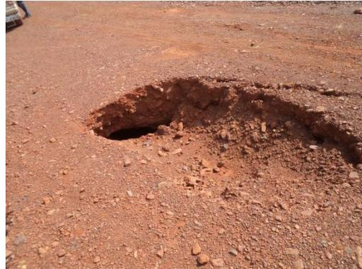
Fig. 5– Sink hole in the embankment
