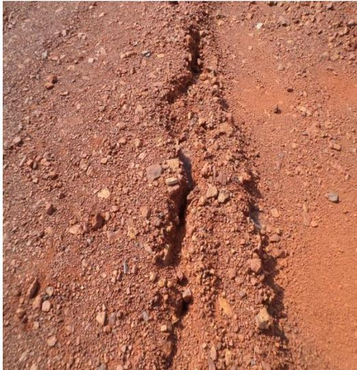
Fig. 4– Longitudinal crack in the embankment
