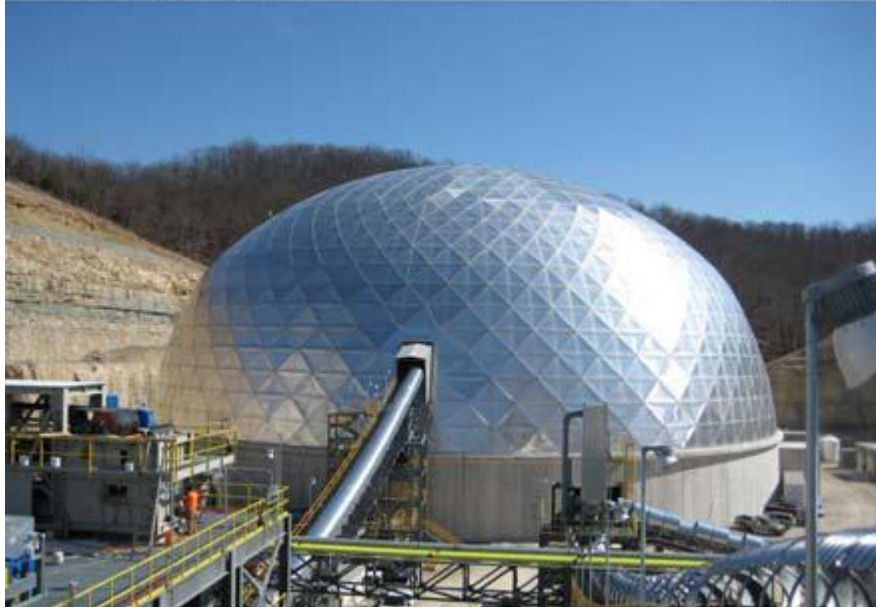
Fig. 4 Dome shaped covered structure for the coal stockpile
