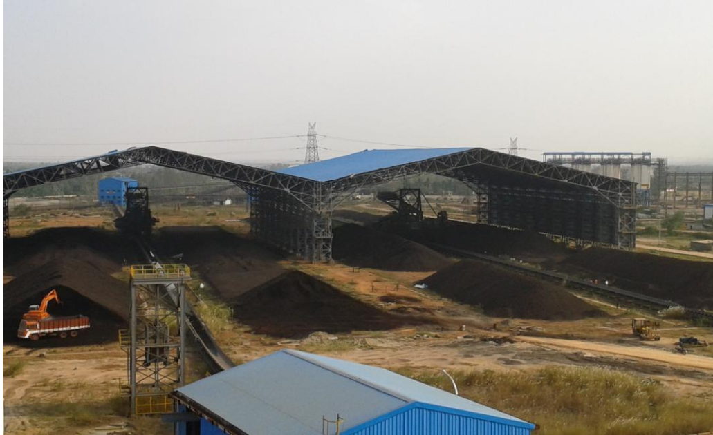
Fig. 3 Covered storage shed for the conventional coal stockpile
