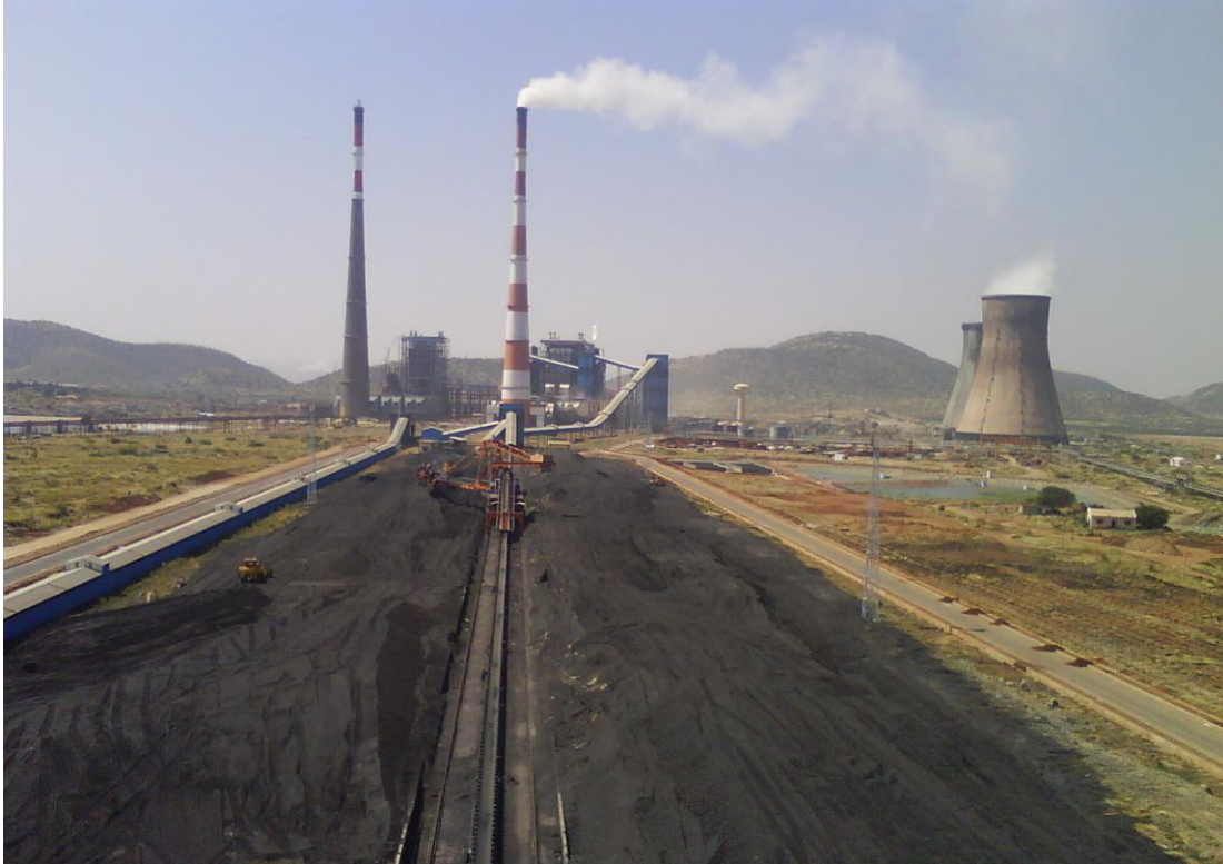
Fig. 1 Typical coal stockpiles in a Thermal Power Plant
