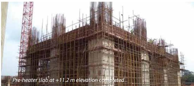
Pre-heater slab at +11.2 m elevation completed
