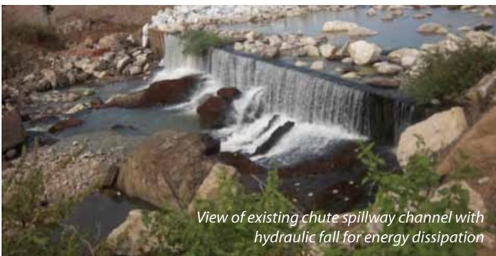
*View of existing chute spillway channel with hydraulic fall for energy dissipation*
