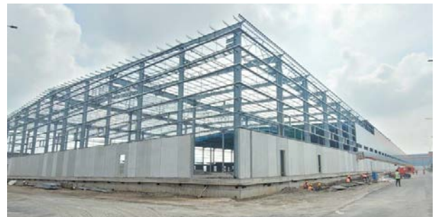
Figure: Usage of Prefabricated Wall Panels for building enclosure
